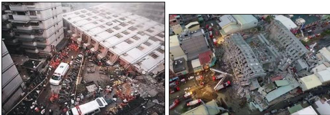
(b) RCC buildings (Taiwan earthquake, 2016 (NDTV, 2016))
