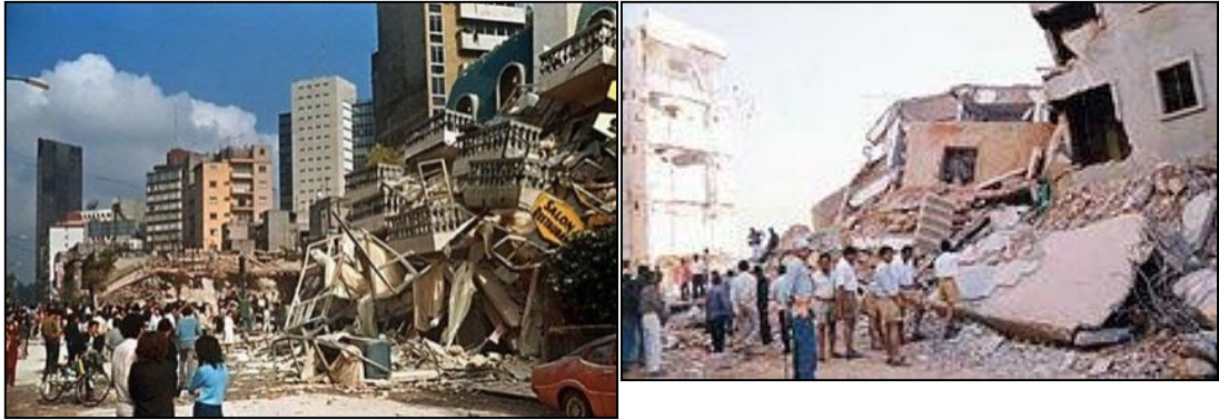
(a) URM buildings (Bhuj Earthquakes 2001, India (Singhania, 2016))
