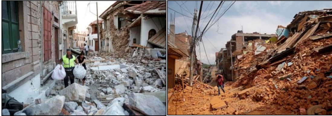
(a) URM buildings (Nepal earthquake, 2015 (Masood, 2015))
