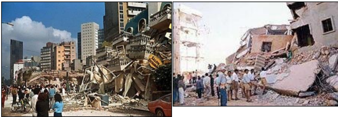
(a) URM buildings (Bhuj Earthquakes 2001, India (Singhania, 2016))
