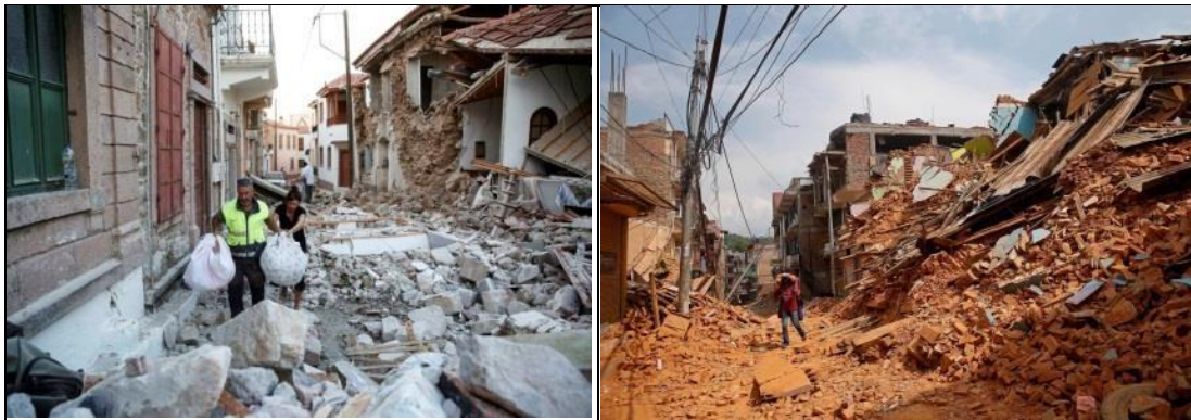
(a) URM buildings (Nepal earthquake, 2015 (Masood, 2015))
