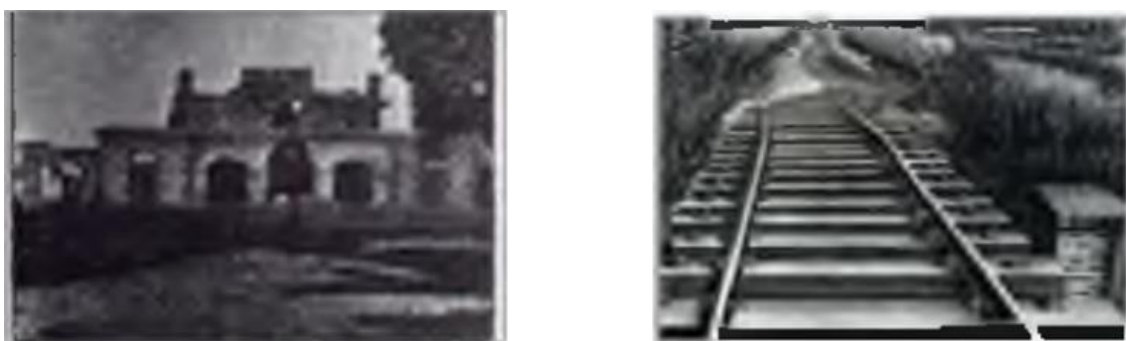
Figure 1.5: Damage of building in 1897 earthquake and damage of rail track in 1997 earthquake
