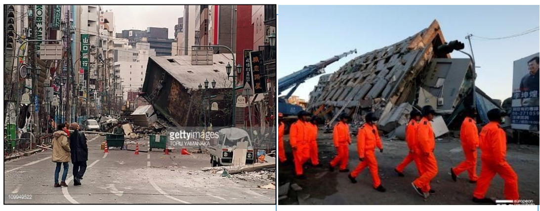
(b) RCC building first condition (Great Hanshin Earthquake 1995, Japan (Yamanaka, 1995))
