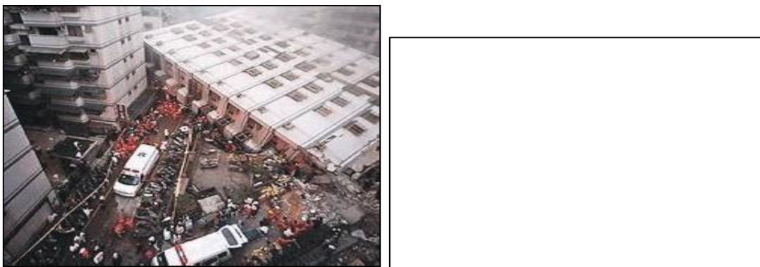
(b) RCC buildings (Taiwan earthquake, 2016 (NDTV, 2016))
