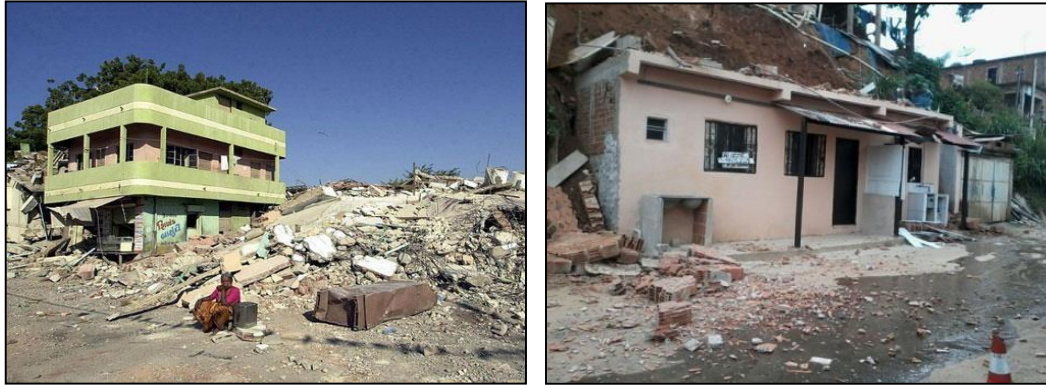
(b) RCC buildings (Bhuj Earthquakes 2001, India (Datta, 2001))
