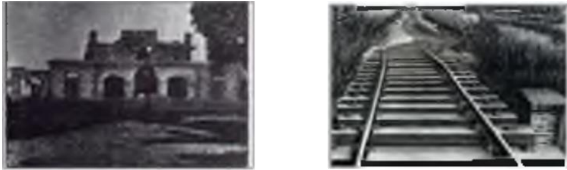
Figure 1.4: Damage of building in 1897 earthquake and damage of rail track ink 1997 earthquake in Rangpur (Source: Ansary et al. , 2003)
